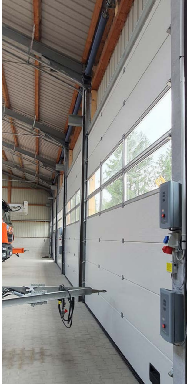
OSP door with lift and roof follower fitting
