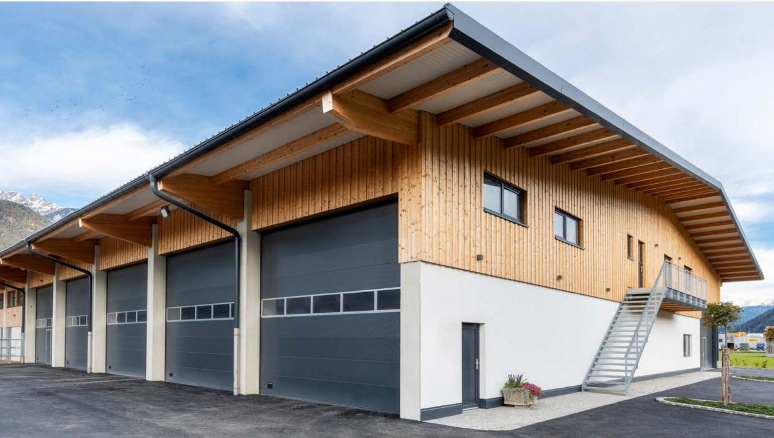
OSP doors in anthracite grey RAL 7016 with light section in natural aluminium
